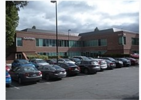
The former MIPS Technologies building in Santa Clara
